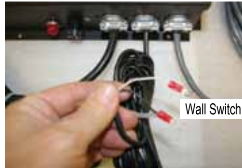
Figure 11. (Remote Switch Wire connection)
