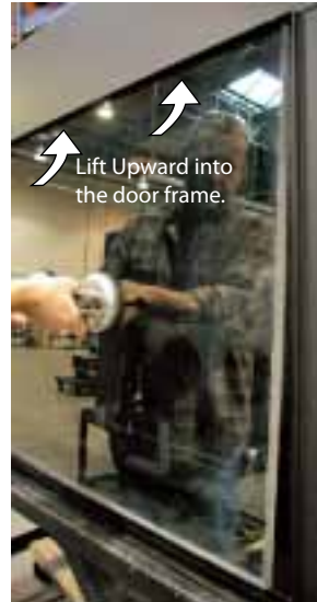
Figure 17c. (Lift the door upward)
