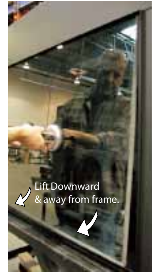
Figure 17d. (Lift the bottom of the door outward)
