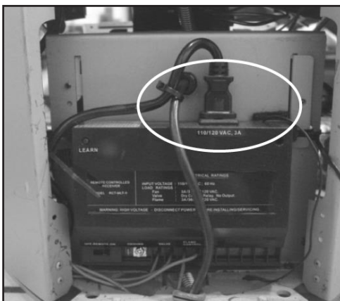
Figure 8.31 Plug the 2-prong blower cord directly into the 3-prong polarized plug on the back of the receiver. This receptacle output is 110/120 VAC, 3 AMP.
