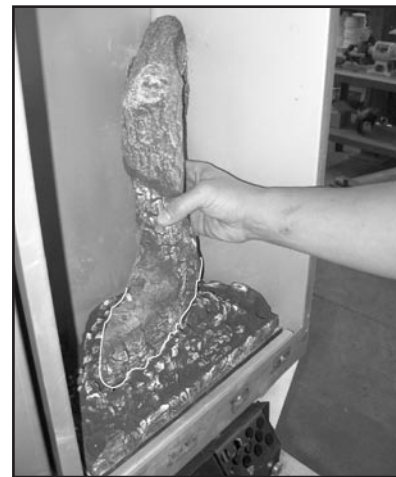
Figure 8.16 Place log #1 into the cradle in the burner. Lean the log back towards right corner of firebox.
